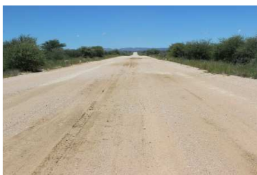
Existing road to Omburu Substation
