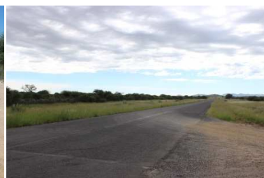
Existing road to Osona Substation
