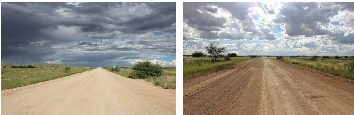
Figure 64 | MR29 access road to the proposed Hardap PV site
