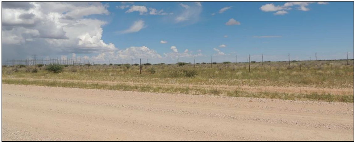
Figure 47 | View of the Hardap Substation as seen from the C29 Gravel Road
